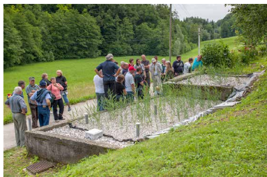
Demonstration sites helped bring the concept of small wastewater treatment plants to life.
